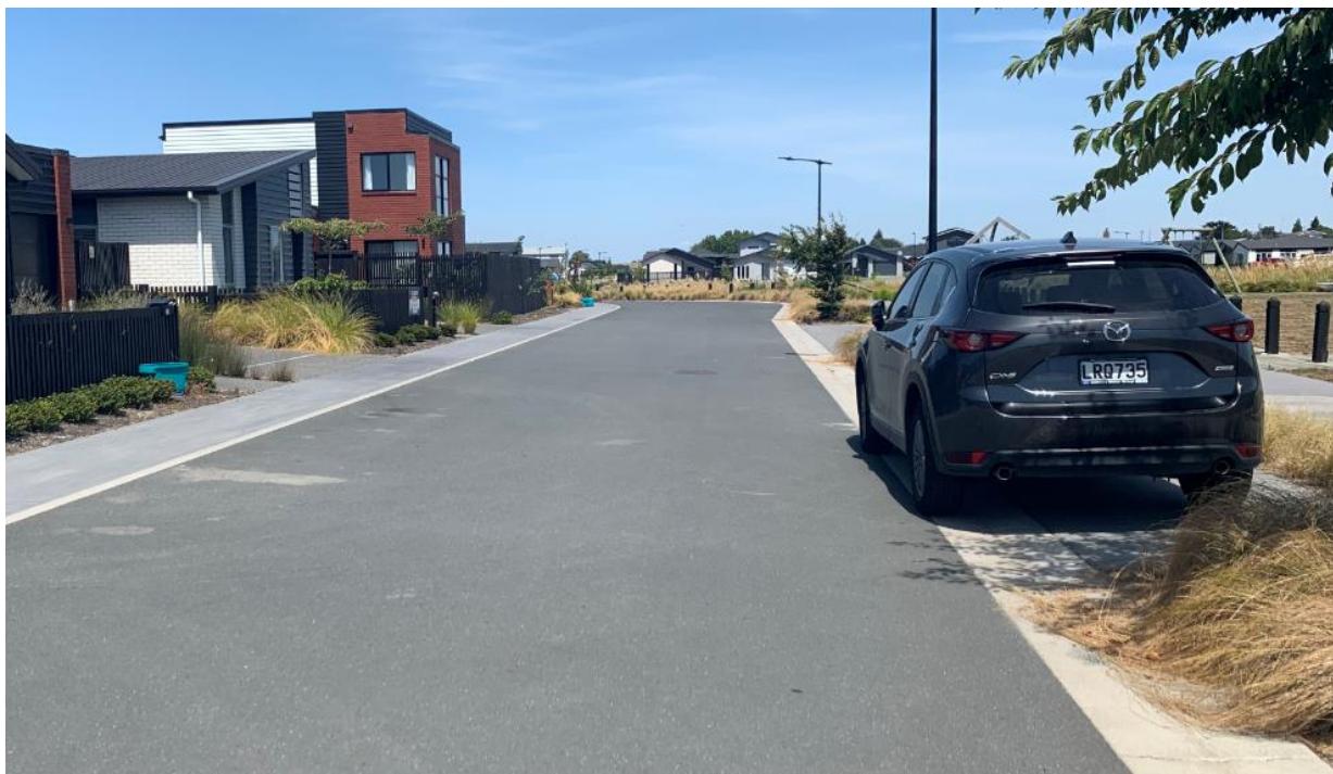
Figure 3: Parallel Parking Encroaching into Movement Lane
