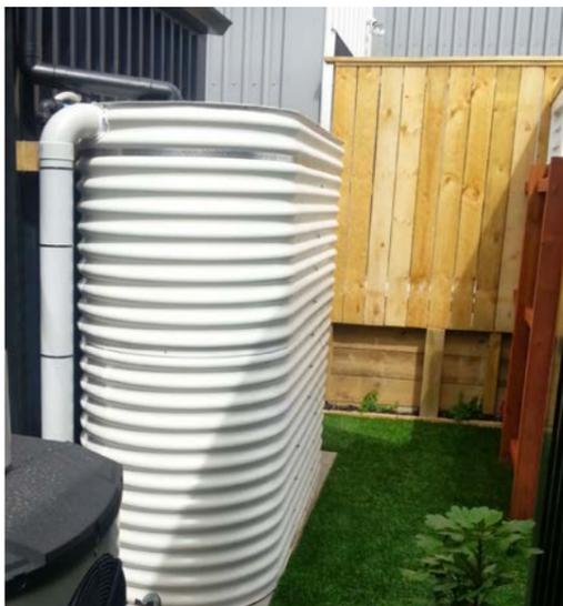
The Detention Tank works by temporarily storing the collected rainwater and then slowly releasing the water through a small outlet in the tank. This storage and slow release of the rainwater reduces the peak stormwater flows during a rainfall event and hence reduces the impacts on downstream infrastructure and/or streams.
