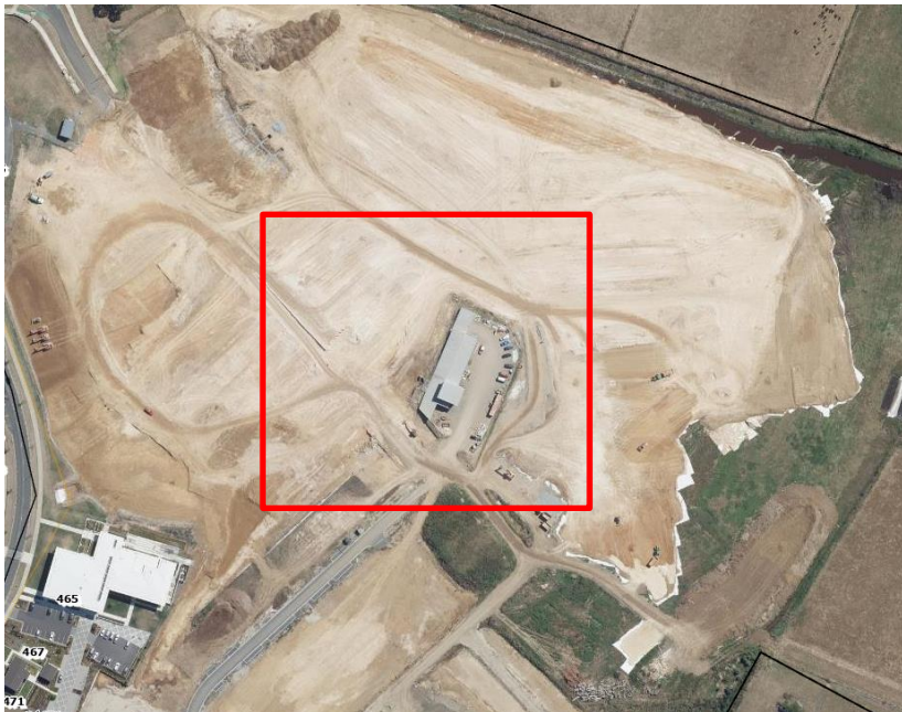
Image 1 – Aerial View of Subject Site with Block Plant outlined in Red
